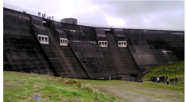
Figure 14. Downstream face showing siphons and sluice gates
