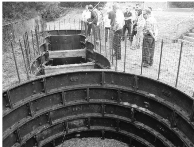
Figure 9. Demonstration section of shafts and trench
