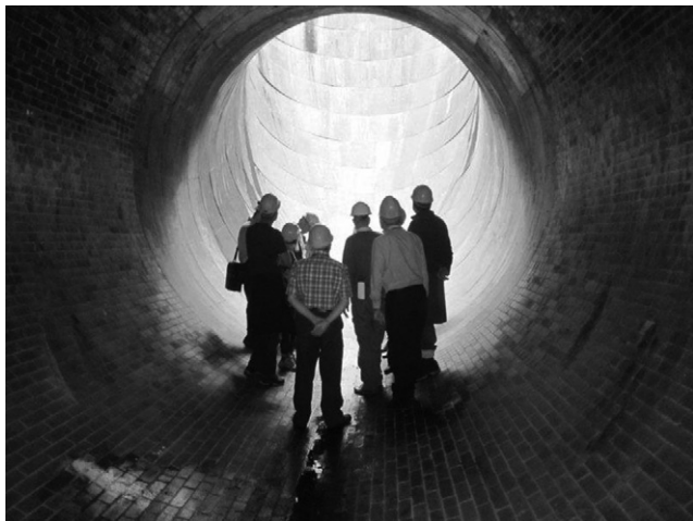
Figure 8. Outlet tunnel from the bellmouth
