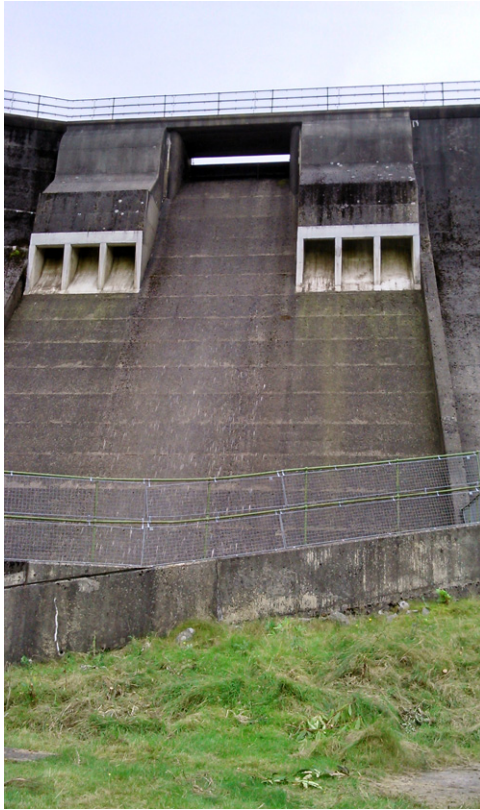
Figure 12. Siphons and adjoining sluice gate
