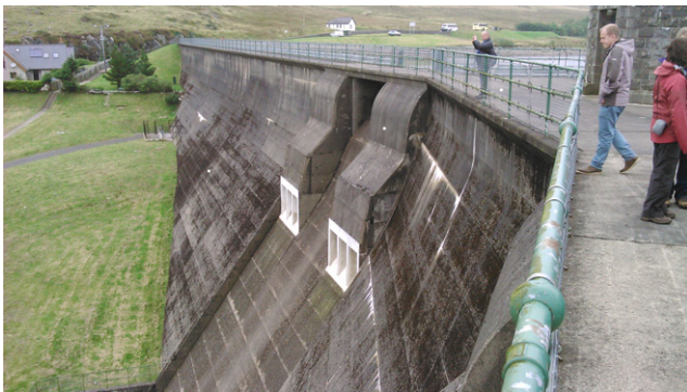
Figure 13. View from dam crest
