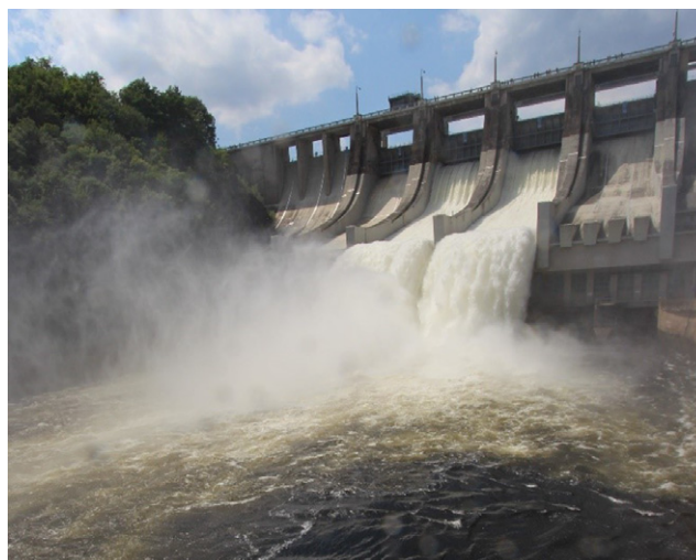
Slapy dam, Czech Republic (photograph: Ian Hope)
