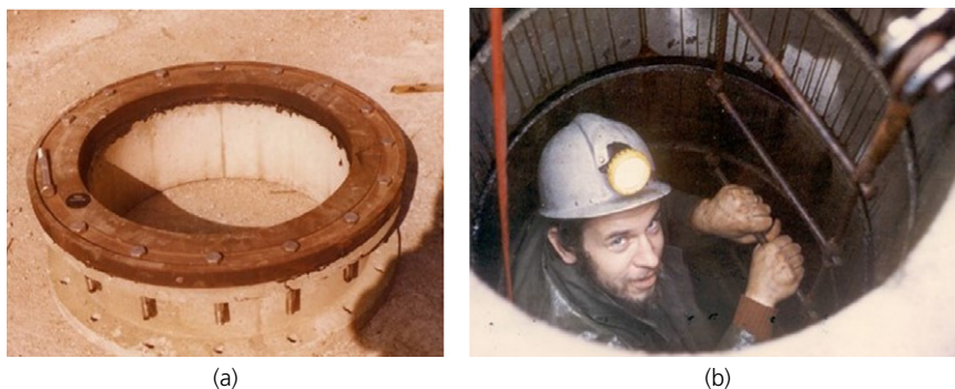
Figure 8. (a) Typical detail of neoprene ring and (b) the decant inspection
