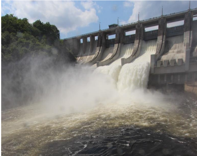
Figure 7 Partial radial gate opening
