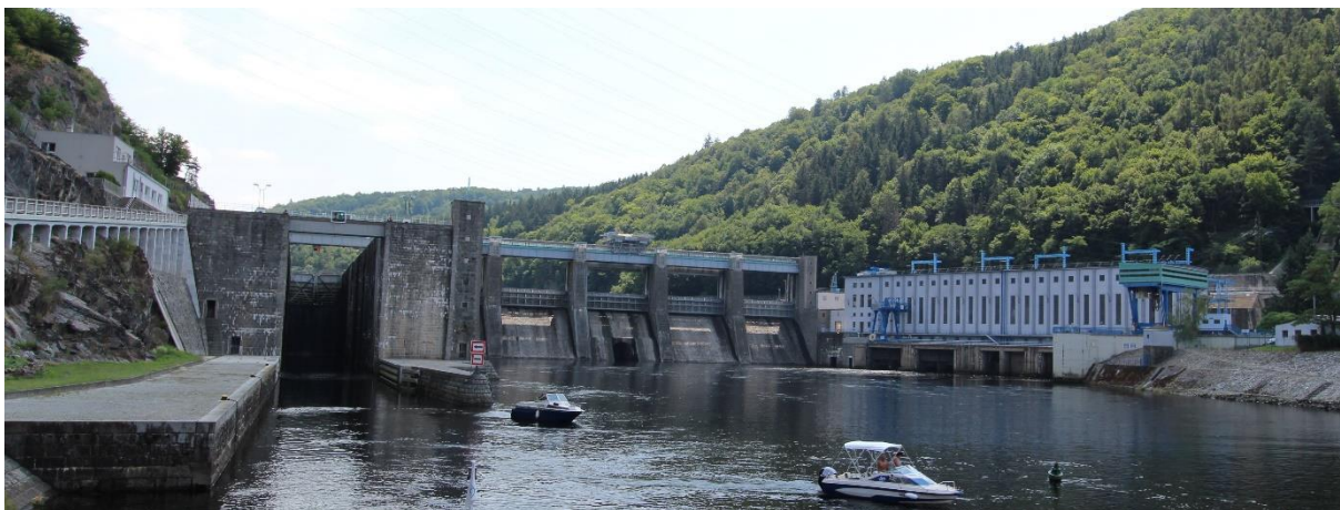
Figure 4 Approaching the Stechovice Dam with lock
