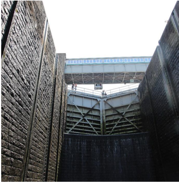
Figure 5 The 20m-high lift within the locks (for scale, note the spectators on the gate)
