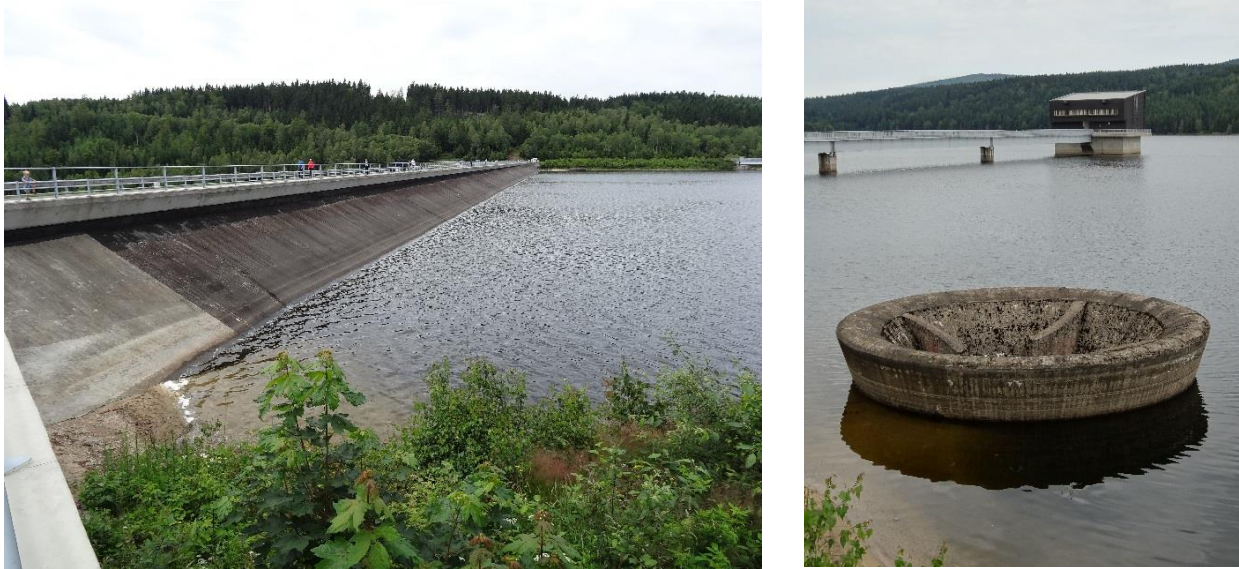
Figure 9 Josefov Dul dam and spillway shaft
