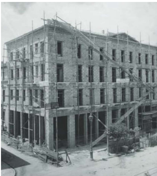
Figure 1. Majestic Hotel (1925) showing robustness of members and eclectic design (reproduced from The Civil Engineer Andreas K. Drakopoulos , p. 270)
