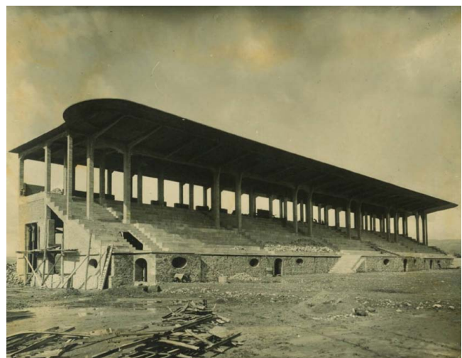
Figure 3. The canopy of the Hippodrome of Athens (1924) (reproduced from The Civil Engineer Andreas K. Drakopoulos , p. 221)
