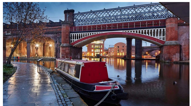
Figure 1. Castlefield Viaduct, Manchester, UK (courtesy of National Trust)
