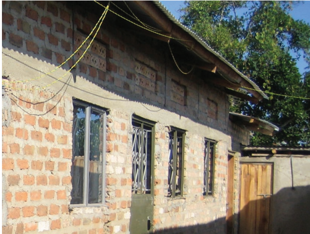
Figure 2. Permanent ventilators on windows and doors
