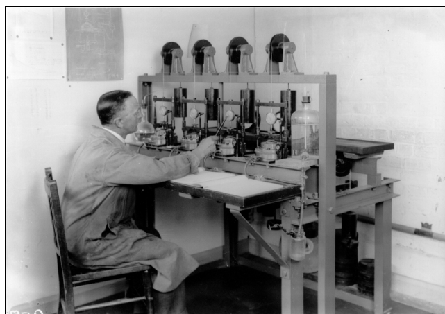
Fig. 2. Set of four oedometers
