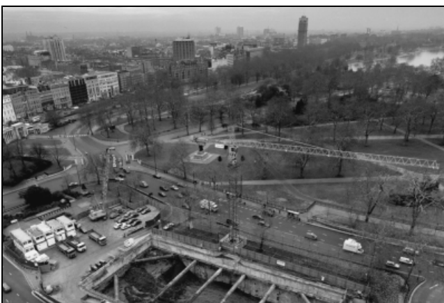
Fig. 1. Typical propped excavation (courtesy of Bachy Soletanche Limited)
