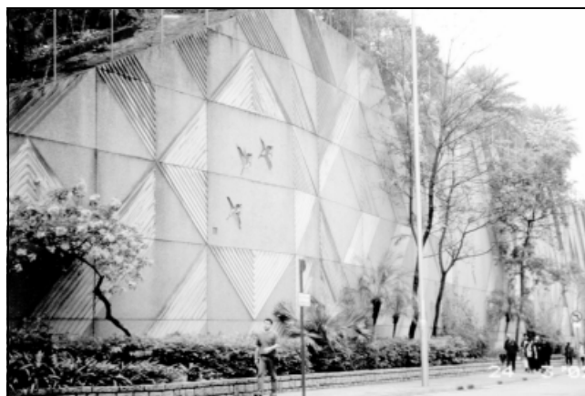
Fig. 2. The blend of toe planting and the design of the surface panels provides both greenery and a harmonious appearance to this 11 m high retaining wall
