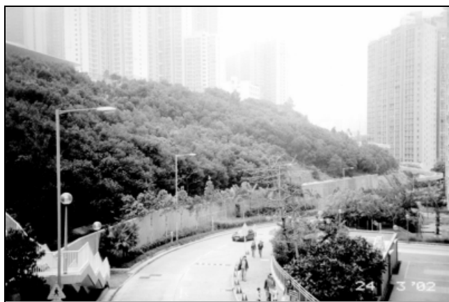
Fig. 1. Planting of shrubs and turfing at the toe and crest of retaining walls naturally integrates the man-made slope features
