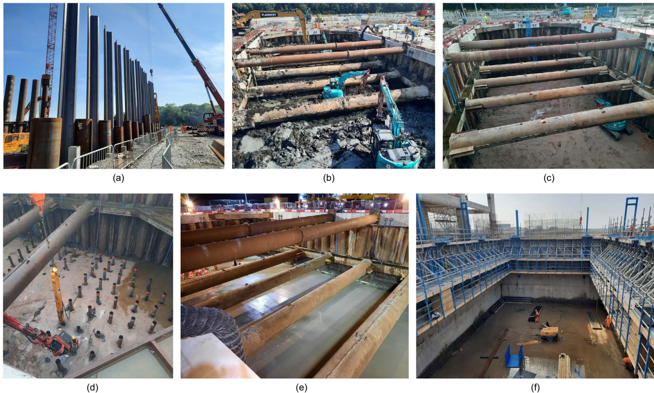
Fig. 5. Photographs of the excavation and bunker structure during construction: (a) stage 2; (b) stage 8; (c) stage 10; (d) stage 11; (e) stage 12; (f) stage 17
