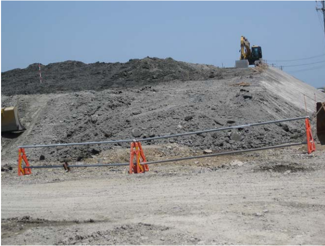
Figure 9. Extra fill on revetments using MDC lumps in 2011
