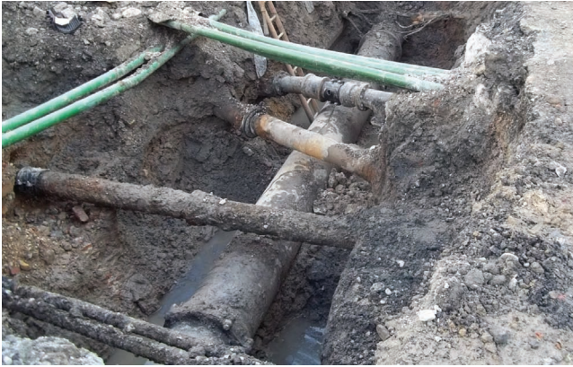
Figure 7. An exposed 20 in. (0.508 m) trunk main in situ at Regent Street in central London with several other pipes and services crossing it, showing the restricted space available around a main
