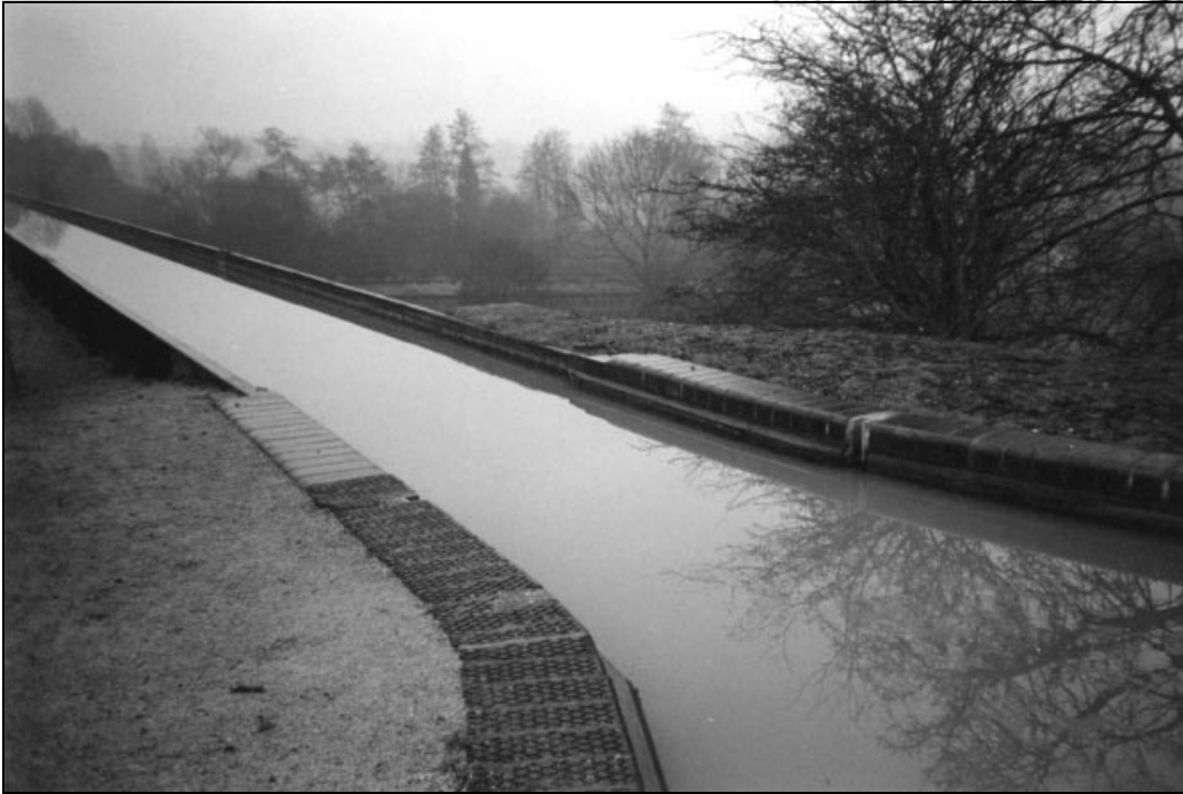
Fig. 1. Edstone Aqueduct—sympathetic restoration
