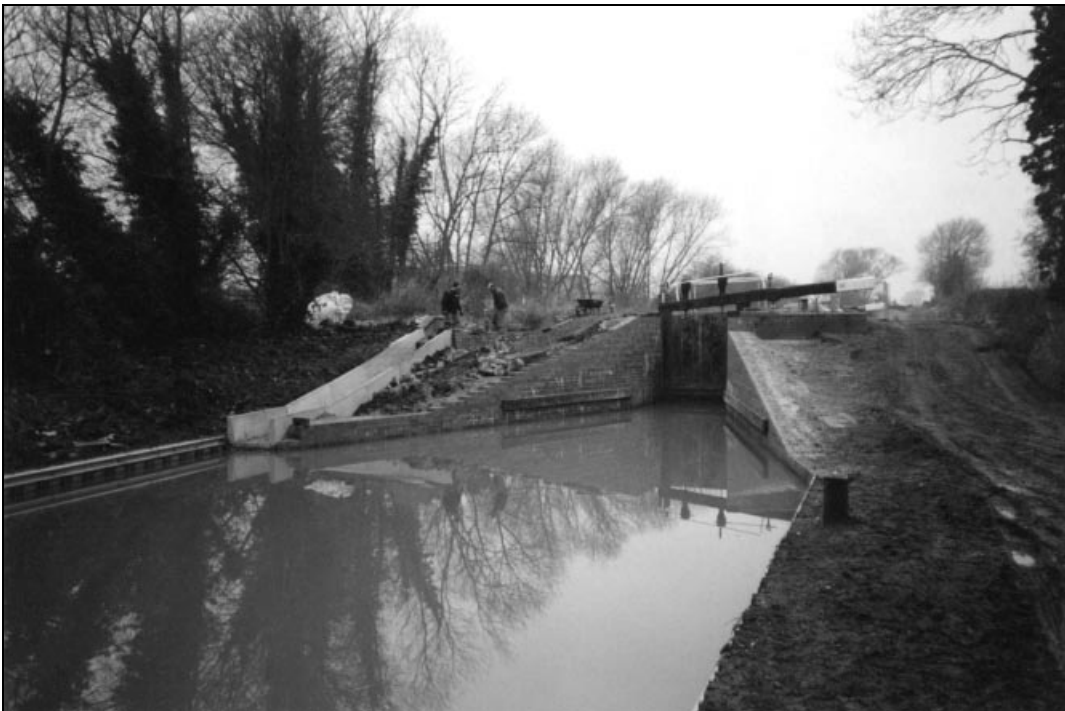
Fig. 8. Major repair of lock walls (lock 50)
