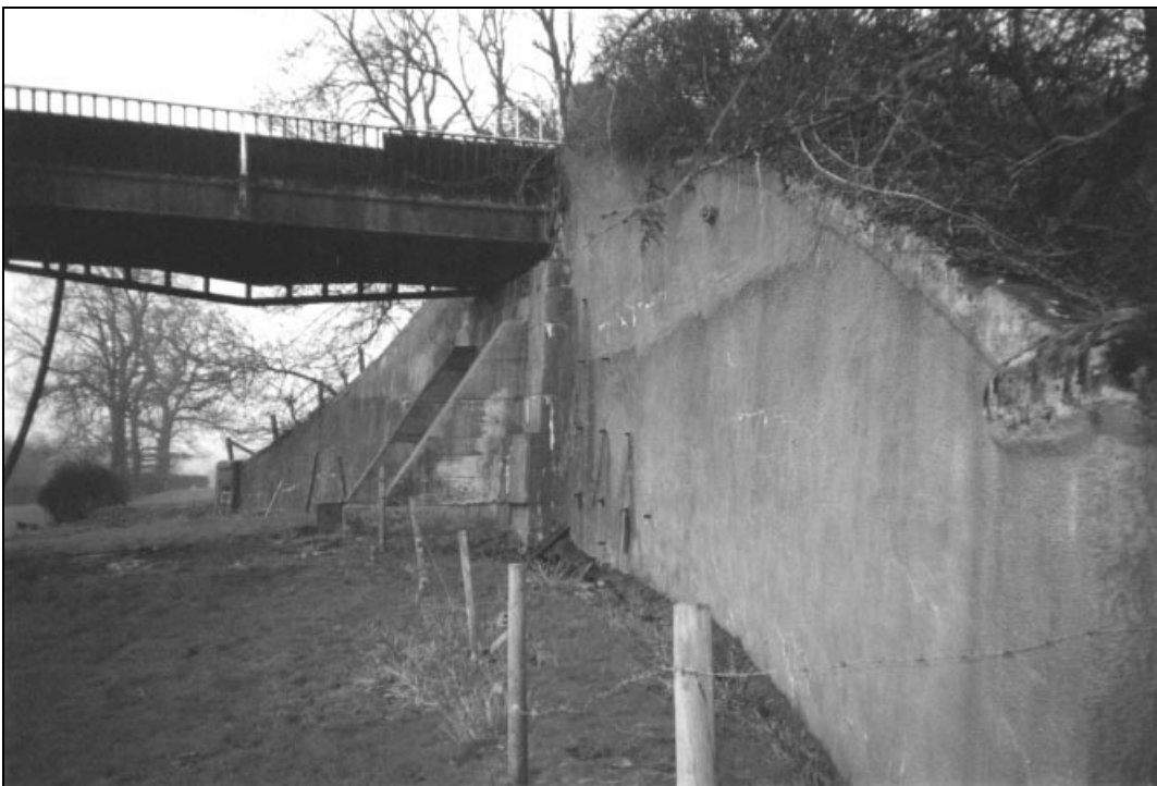
Fig. 2. Edstone Aqueduct—non-sympathetic restoration
