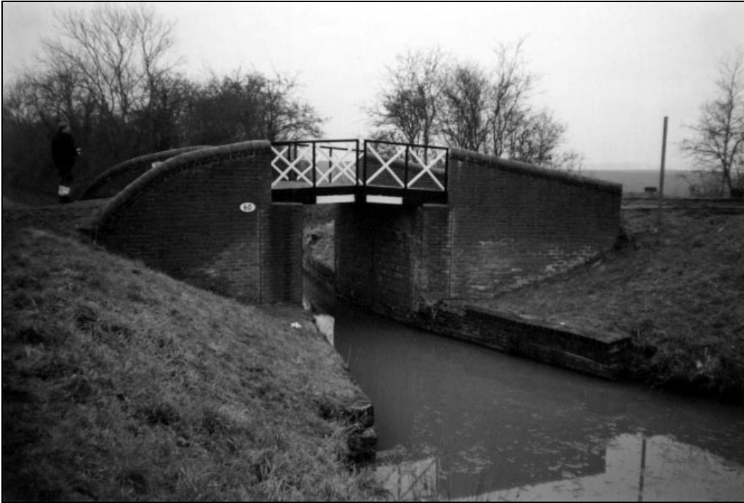
Fig. 5. Packhorse bridge—substantial rebuild
