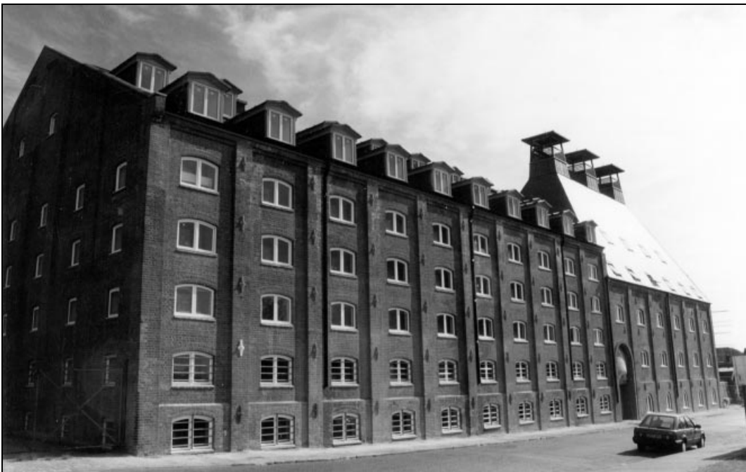
Fig. 2. Felaw Maltings following restoration work
