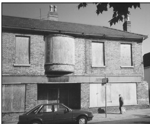
Fig. 1. No. 90 Risbygate Street before restoration
