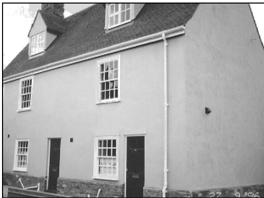
Fig. 4. No. 96a and 96b Risbygate Street following restoration
