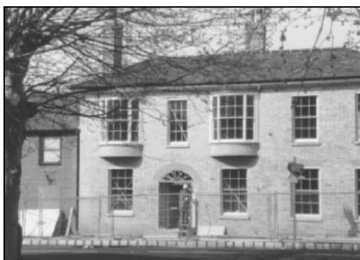
Fig. 2. No. 90 Risbygate Street following restoration
