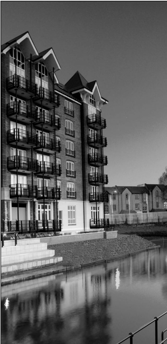
Fig. 11 Building on the water's edge required careful design, particularly with regard to basement car parking. Here, a naturally formed volclay mat protects the car park from water ingress
