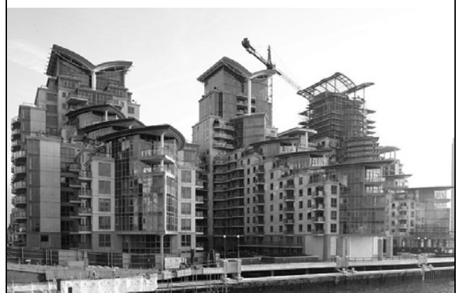
Fig. 4 River-wall repairs and working adjacent to the river
