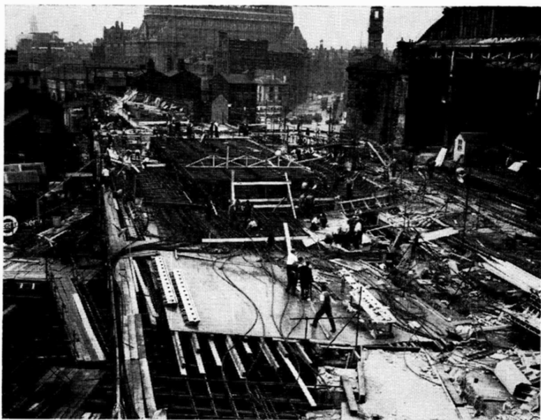
FIG. 18.—FAIRFIELD STREET BRIDGE AT AN EARLY STAGE
