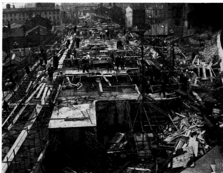
FIG. 19.—FAIRFIELD STREET BRIDGE AT AN ADVANCED STAGE
