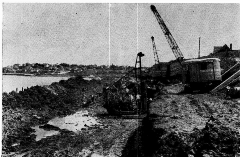
FIG. 28.—HERNE BAY, STUDD HILL, WORK IN PROGRESS BEHIND CLAY BANK
