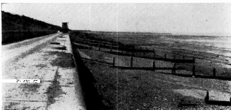
FIG. 31.—HERNE BAY, STUDD HILL, WORK NEAR COMPLETION SHOWING GROYNES HOLDING SHINGLE BEACH
