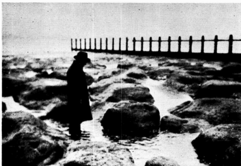
FIG. 25.—FORESHORE SCOUR BETWEEN SELSEY AND BRACKLESHAM
