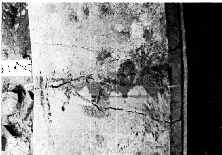
FIG. 60.—SAME SECTION AS IN FIG. 59, WITH CONCRETE TOPPING AFTER TESTING
