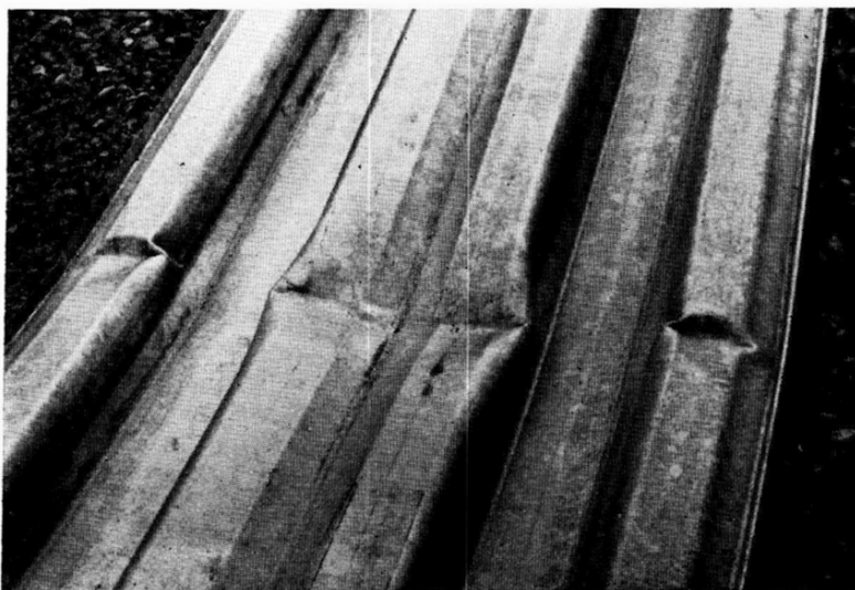
FIG. 59.—RE-ENTRANT SECTION IN BUCKLED FORM AFTER LOADING TO DESTRUCTION
