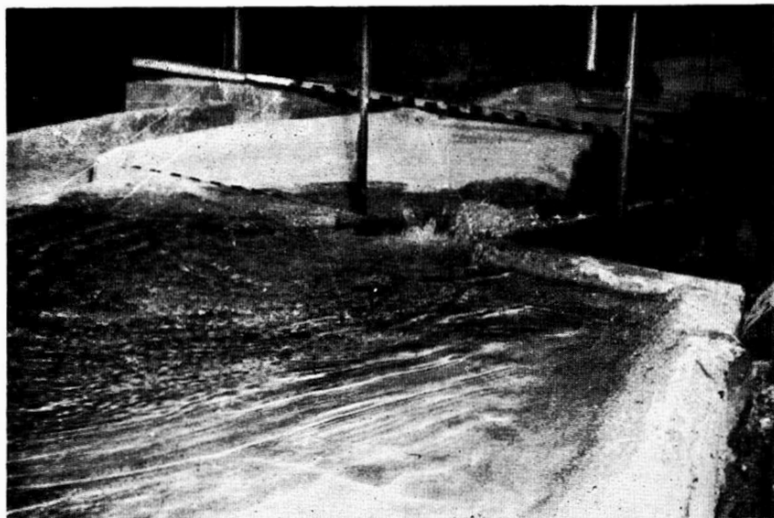
FIG. 39.—VIEW FROM THE EAST OF A DISCHARGE CORRESPONDING TO 13,000 CUSECS THROUGH THE BELLMOUTH CONSTRUCTED TO THE RECOMMENDED DESIGN. HYDRAULIC JUMP RISES ABOVE THE CHANNEL WALLS ONLY AT THE CENTRE
