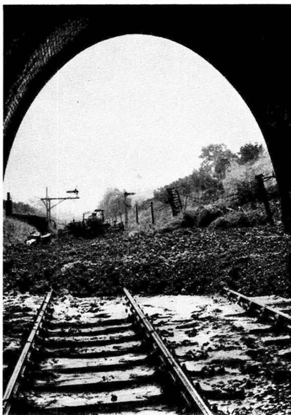
FIG. 58: SEVENOAKS TUNNEL SOUTH FACE LOOKING OUT FROM TUNNEL—CLEARING IN PROGRESS
