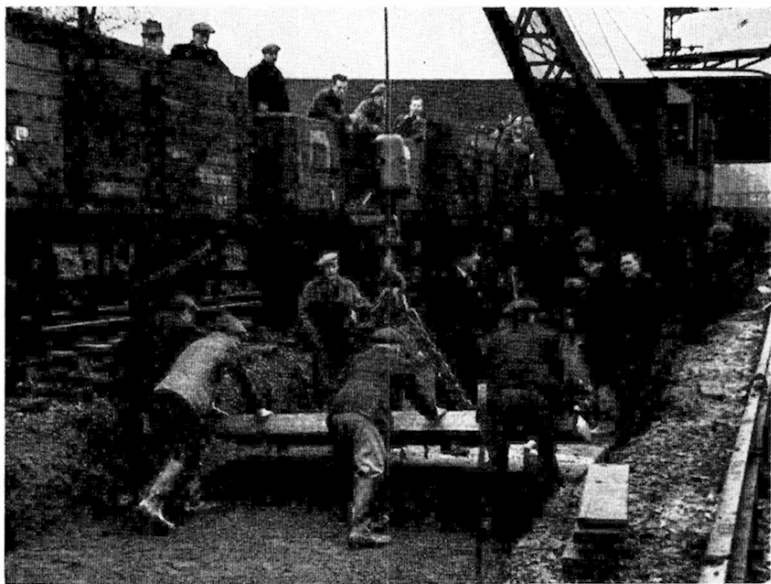
FIG. 54: FORMATION BLANKETING OF LONDON CLAY AT CLAPHAM JUNCTION USING "ONE-PIECE" SLABS—STILL FUNCTIONING WELL
