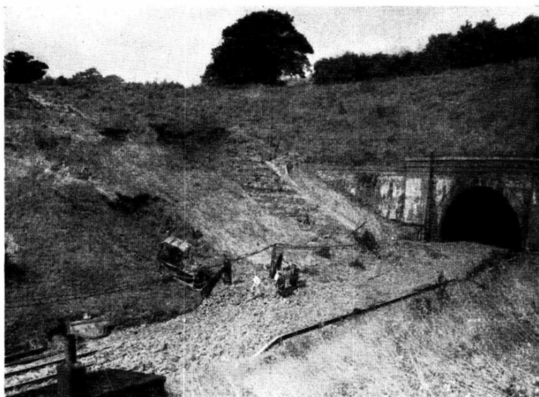
FIG. 56: SEVENOAKS TUNNEL SOUTH FACE—EARTH SLIP IN CUTTING 5 SEPTEMBER, 1958
