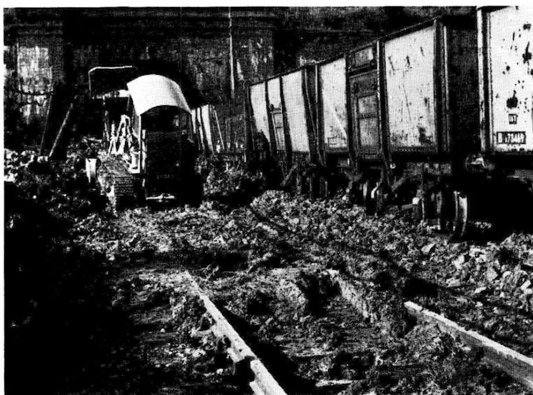
FIG. 57: SEVENOAKS TUNNEL SOUTH FACE—CLEARING "PORRIDGE"
