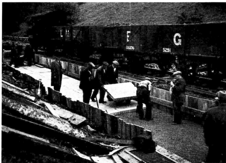
FIG. 53: 1938 FORMATION BLANKETING OF WEALD CLAY USING SMALL SLABS—FAILED AFTER 22 YEARS
