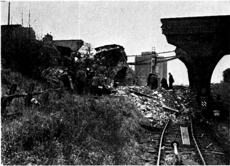
FIG. 45: ASPINAL ROAD BRIDGE—COLLAPSE OF TWO ARCHES DUE TO SUDDEN SLIP
