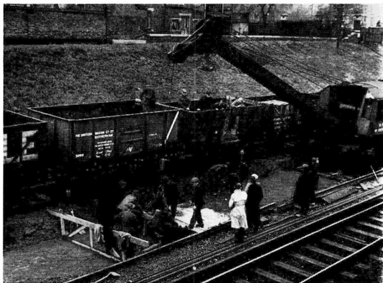
FIG. 55: GENERAL VIEW OF "ONE-PIECE" FORMATION BLANKETING AT CLAPHAM JUNCTION
