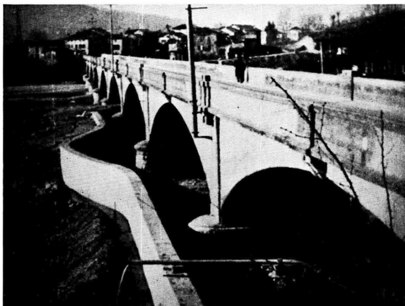
FIG. 50: COFFERDAM PROTECTING FOUNDATION TO OLD BRIDGE AT BUSCHE POWER STATION INTAKE
