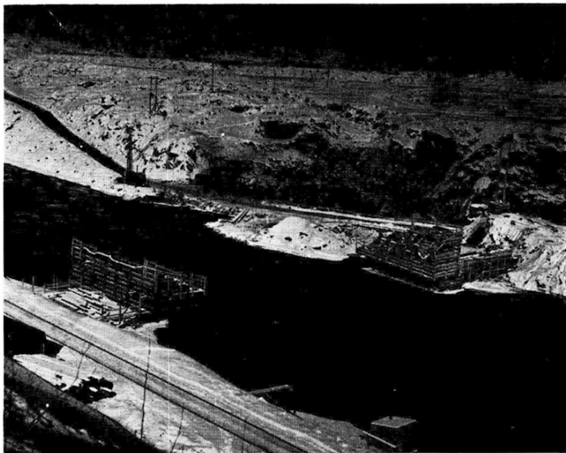
FIG. 53: ST MAURICE RIVER, BEAUMONT DEVELOPMENT. UPSTREAM COFFERDAM, TIMBER CRIBS BEFORE LAUNCHING
