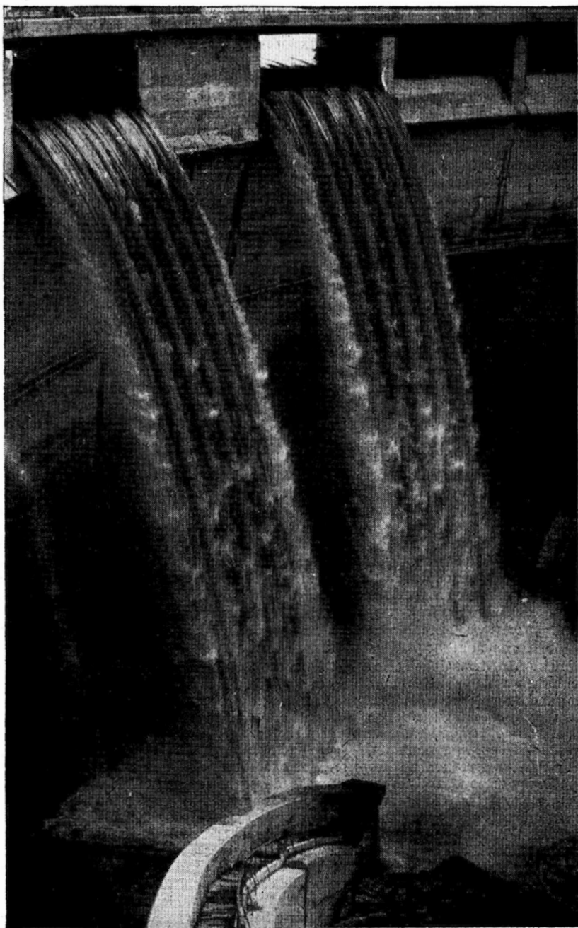
FIG. 40: CENTRE GATES SPILLING AT MONAR DAM
