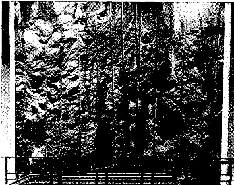
FIG. 34: SMOOTH BLASTING USED IN TRIMMING BASE ROCK WALLS IN THE POWER STATION
