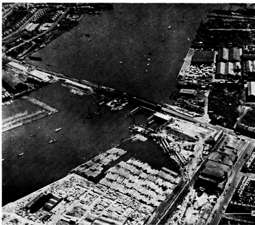
FIG. 17. AERIAL VIEW SHOWING AREA OF CONSTRUCTION YARD
