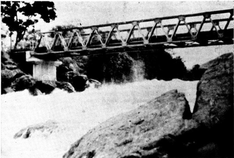
Fig. 20. Callender-Hamilton Bridge over the Shire river
