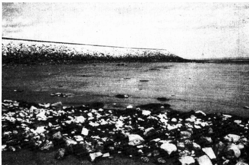
Fig. 9. Completed length of sea wall with stone pitching and concrete wave return wall
