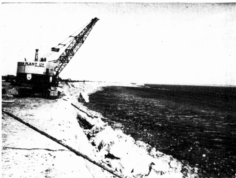
Fig. 8. Stone blocks being placed as armouring to sea wall, fronting the Welsh Grounds
