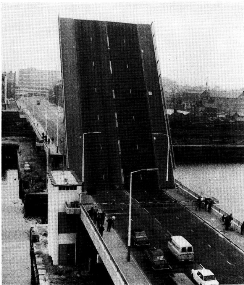
Fig. 30. The Michaelson Bridge
