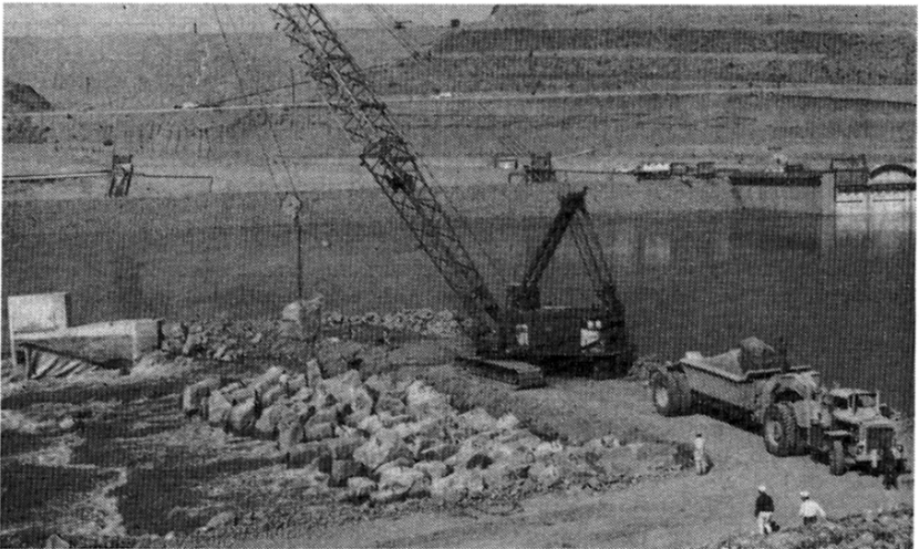
Fig. 15. Armoring downstream slope of left-hand rock weir. Note access over gabions, and end of bag in foreground ; also rocks washed over bag 3, centre left
