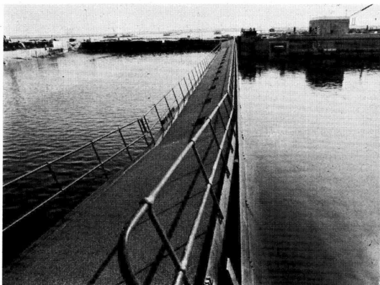
Fig. 4. Trial opening of dock gate
