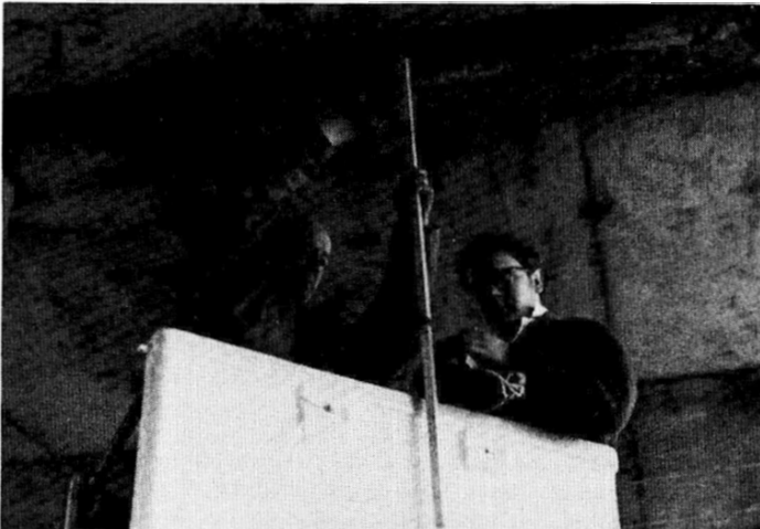
Fig. 13. Taking reinforcement potentials inside an expansion joint gap
