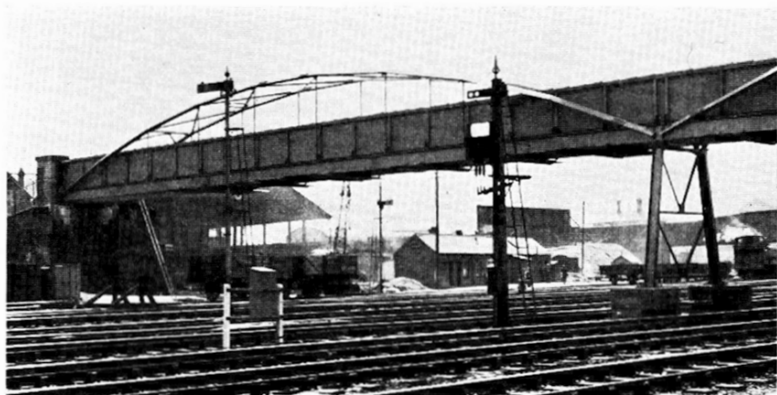
FIG. 19.—100-FT TIED-ARCH SPAN OF FOOTBRIDGE NEAR CARDIFF
