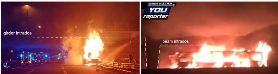
Figure 5. Pictures showing the flame height in the fully developed stage of the fire
