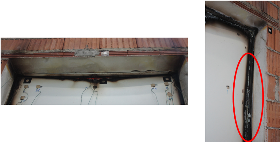
Figure 21. Observed gap formation during the fire resistance test at the upper edge of the door (left) and burning marks above the door lock after the test (right)
