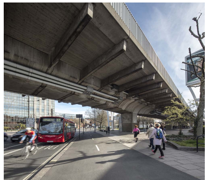
Figure 3. Photograph of the Hammersmith flyover at street level below the bridge. Photograph reproduced with the kind permission of Ramboll UK
