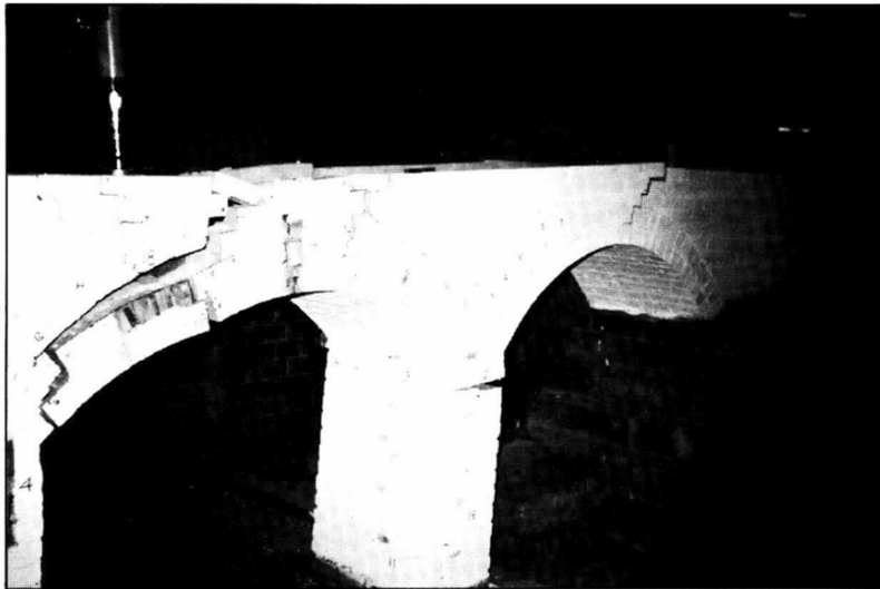
Fig. 19. Model multi-span bridge test
