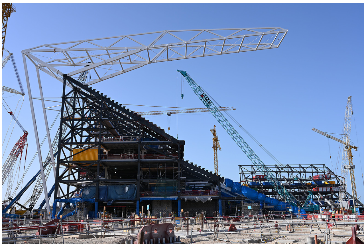
Figure 10. Roof structure during installation
