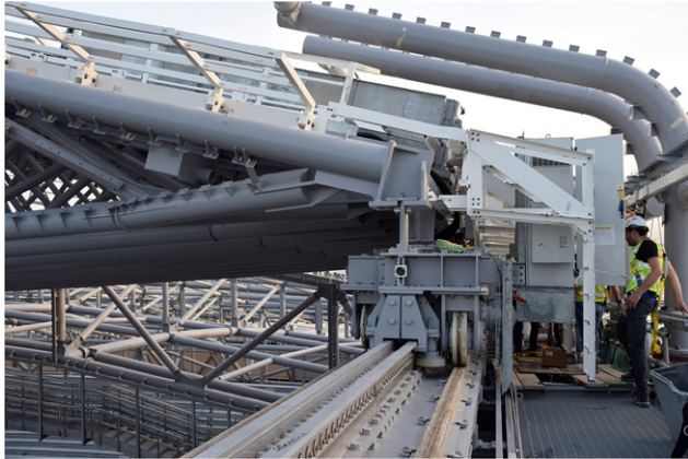
Figure 13. Driving carriage with rail structure of retractable roof during commissioning
