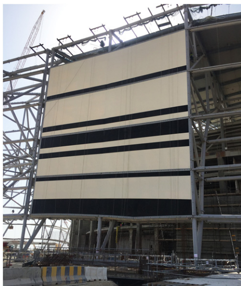
Figure 2. Construction stage of facade membrane
