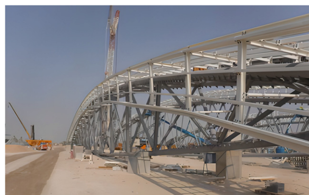
Figure 12. Retractable roof truss assembly stage
