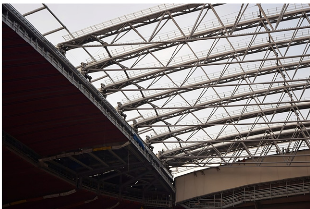
Figure 14. Moving trusses with spreader arms before membrane installation
