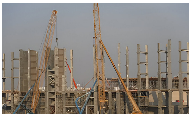
Figure 3. Installation of precast concrete columns
