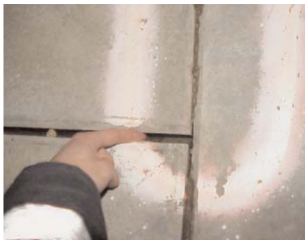
Figure 13. Examples of irregularities in the segmental supports. Uneven supports might cause cracking.
