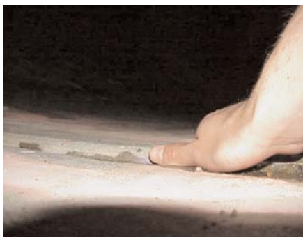
Figure 13. Examples of irregularities in the segmental supports. Uneven supports might cause cracking.
