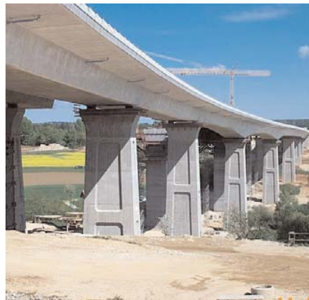
External prestressed bridge designed by Josef Eibl
