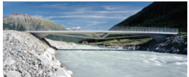
Special Mentions, Civil Engineering Category: Flaz River Bridge, Switzerland; New Svinesund Bridge, Norway/Sweden; Infante Dom Henrique Bridge, Portugal
