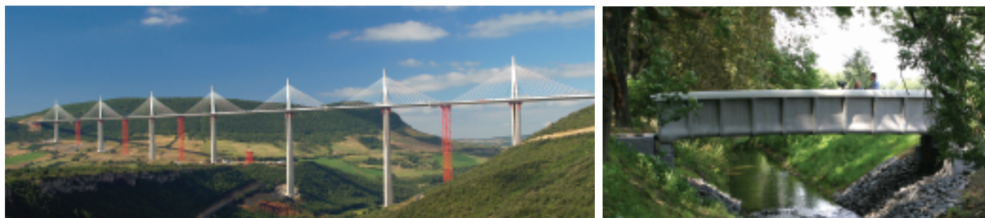
Structures that received "Exceptional Recognition" citations from the Jury: Millau Viaduct, France; Döllnitz Creek Bridge, Oschatz, Germany
