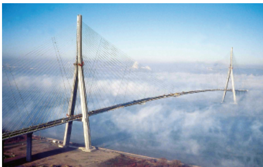
The Normandy Bridge (photo Bouygues Campenon Bernard Group - Vinci)
