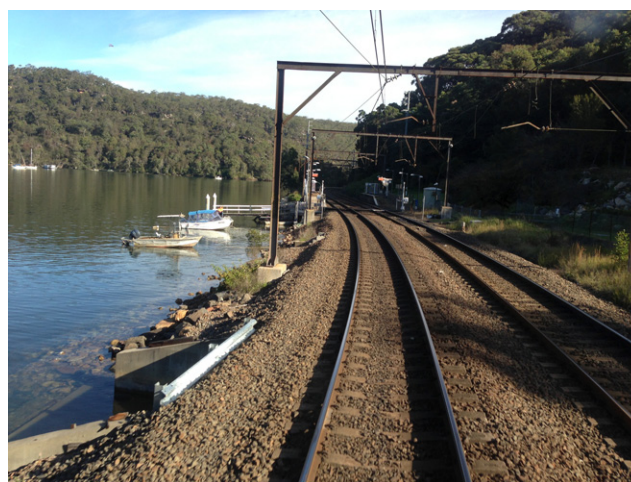
Figure 1. Typical ballast railway track in Australia
