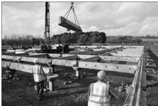
Fig. 2. Use of precast concrete beams at a housing development near Newport in south Wales
