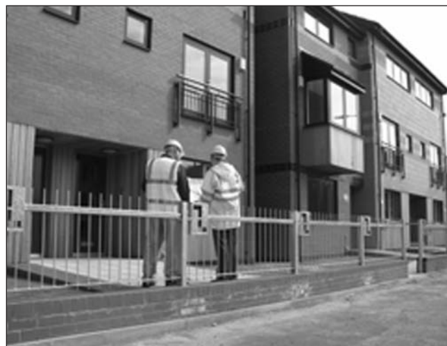
Fig. 4. Completed housing development in Hull, featuring raised floor levels
