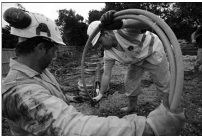
Fig. 3. A heat transfer tube being inserted into a foundation pile
