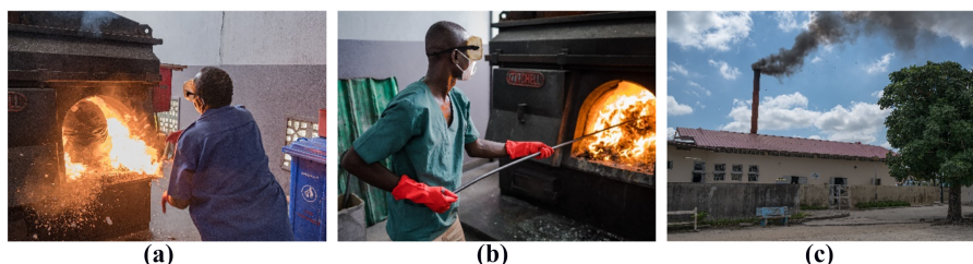
Plate 1. The incinerator installed at BCH, Mozambique, 3 May 2022. (a) A waste operator is manually inserting the fuel into the combustion chamber; (b) a waste operator is manually moving the waste inside the combustion chamber to improve the combustion; (c) the incinerator's chimney and flue gases. Source: Photo by Paolo Ghisu
