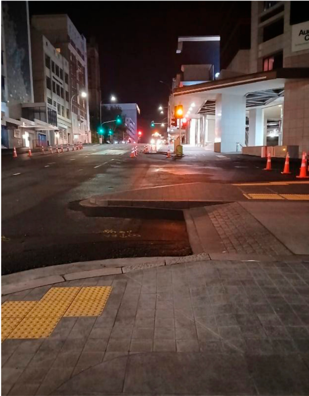
Plate 18. The double entry and sharp curb barriers (construction work in progress)
