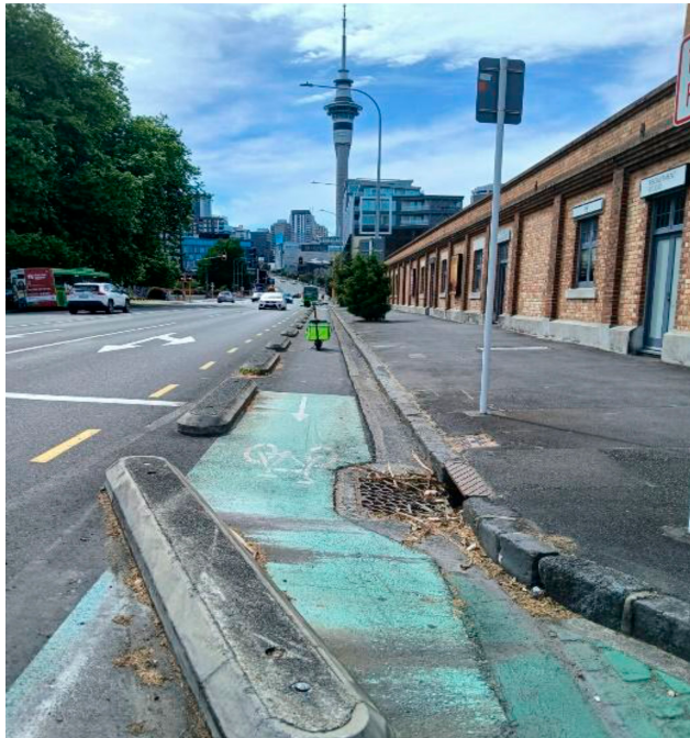
Plate 15. Narrow and interrupted lane near Sky Tower (CBD core), limiting safe scooter turning with an abrupt surface gradient and misaligned markings. Such conditions amplify risk during night-time deliveries
