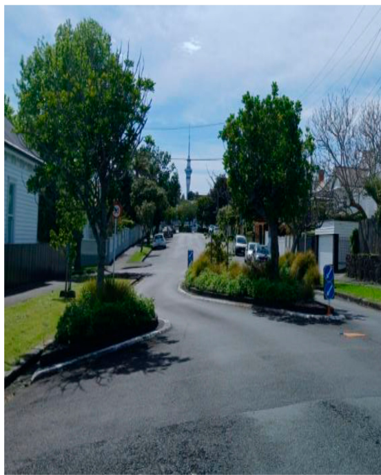
Plate 4. Mid-road tree placement in Ponsonby is creating turning visibility challenges. While promoting sustainability, canopy shadows obscure lane edges
