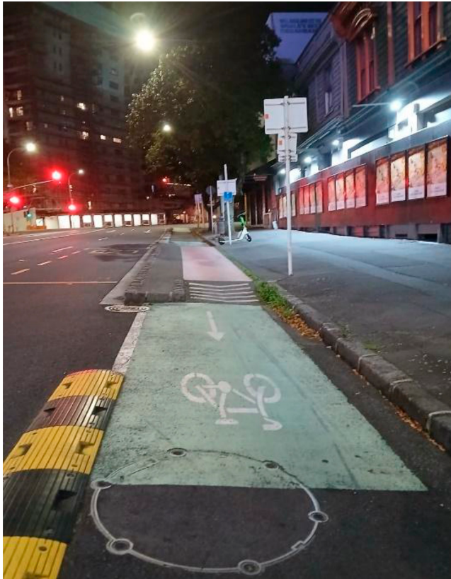
Plate 16. Mid-lane obstacles on the narrow cycle path at Victoria St West. Poor visibility and obstruction placement force unsafe manoeuvres, contradicting Auckland's Smart Mobility objectives
