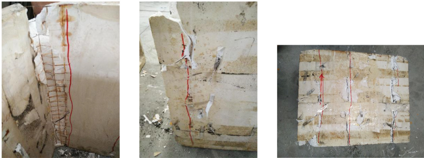
Cross-fault cracked section of lining structure (9#) (c)
