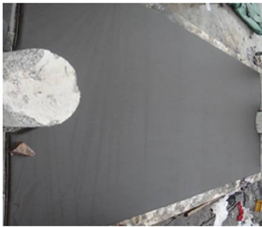
Photo of CA mortar after removing slab
