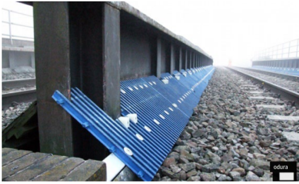
Ballast retaining system for steel beam ballasted deck
