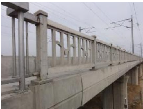
Figure 2. Prefabricated reinforced concrete railings for railway box girders. Source: Internet
